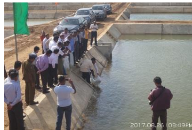
Construction of stage II and fish stocking in Udawalawa Aquaculture Centre
