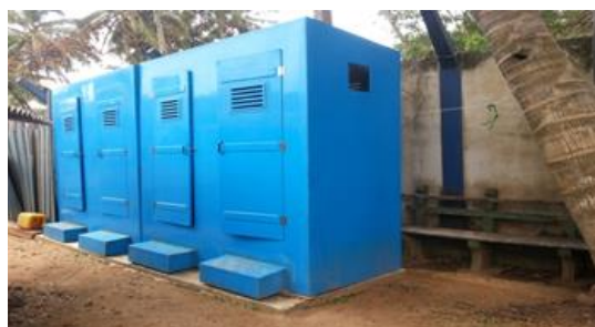
Sanitary facilities of Mirissa Fishery Harbour
