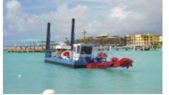
Nil Diyawara Cutter Suction Dredger
