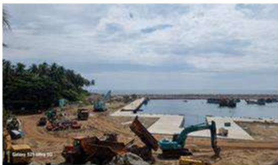
Construction of travel lift bay
