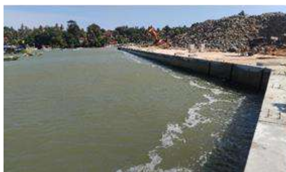
Construction of the platform wall
