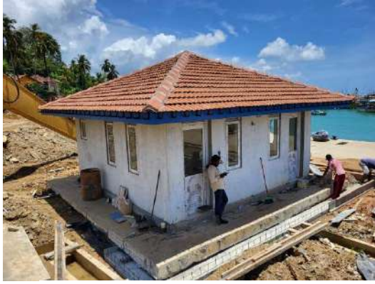
Construction of the fuel office
