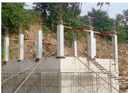
Construction of underground water tank
