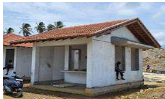
Construction of the Fisheries Office
