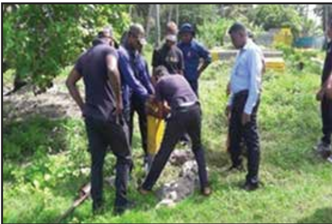
Planting of boundary posts
