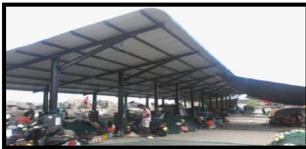
Fully constructed net mending hall
