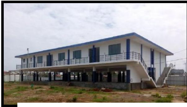
Fully constructed auction hall
