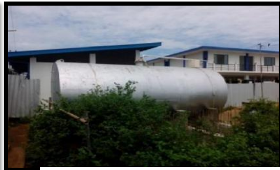
Fuel tank constructed inside the harbour
