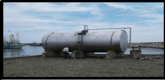
. Renovated Fuel Tank
