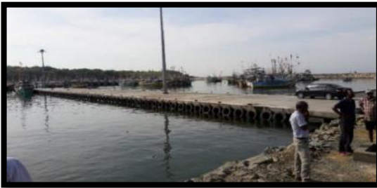
New Service Jetty
