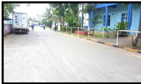
Figure 5.8.7. Renovated internal road system
