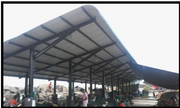
Figure 5.8.3. Fully constructed net mending hall
