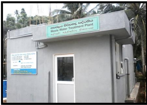
Figure 5.8. 5. Waste water treatment plant
