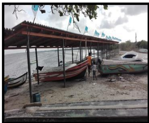
Figure 2.3.1 Construction of multipurpose building at Thiyawarthanwan
