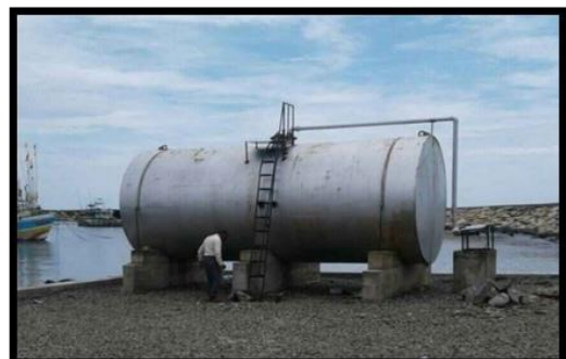
Figure 5.8. 10. Renovated Fuel Tank
