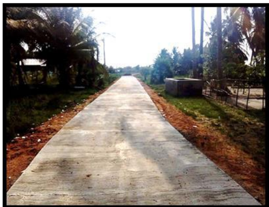
Figure 2.3. 3 Concreting road form Anakutthiya to Manativ Junction
