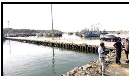
Figure 5.8.9. New Service Jetty
