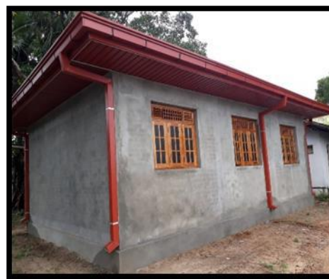
Figure 2.3. 2 Construction of sunshades at Kurakkanhena
