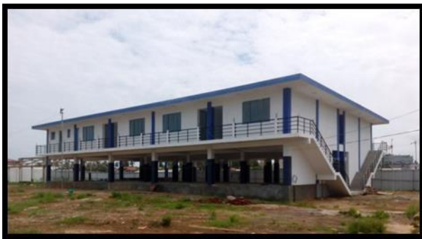
Figure 5.8.1. Fully constructed auction hall
