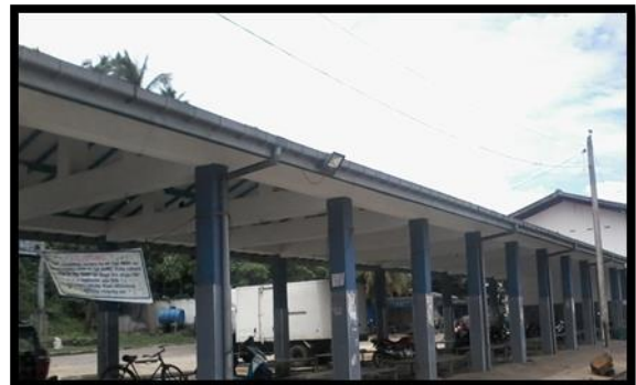
Figure 5.8.4. Constructed new auction hall
