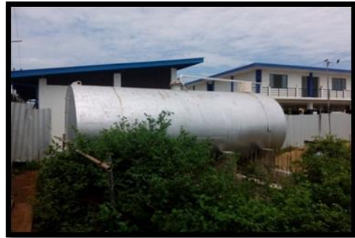
Figure 5.8. 2. Fuel tank constructed inside the harbour
